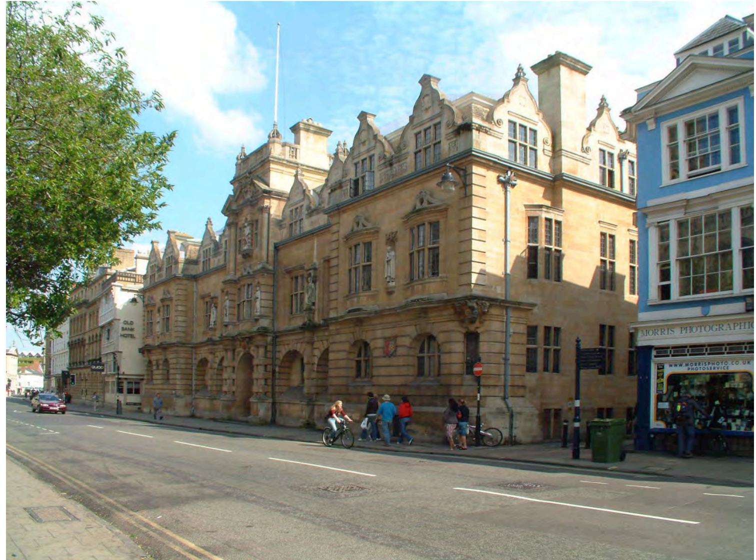
View of Rhodes Building from High Street, looking east
