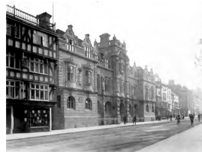
Photograph of Rhodes Building from the High Street, taken in 1912. The photograph clearly shows the railings in front of the College and they appear to be painted a light colour.
